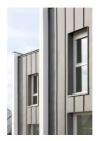
elZinc Natural is a traditional material by excellence. **elZinc® Natural** is the originally metallic grey finish produced by our production process. The natural patina, which develops automatically on exposure to weather, turns the finish to a pleasant mat grey colour.
